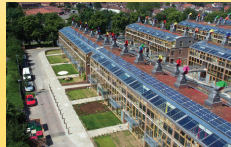
PV on the southern facade of BedZED, UK creates enough electricity for 40 cars
