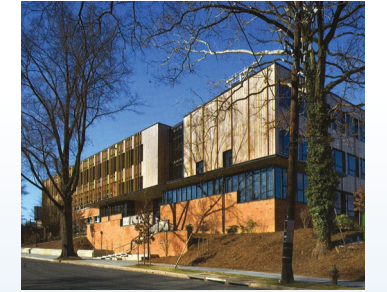
ACTIVE SOLAR CONTROL PANEL SYSTEM
